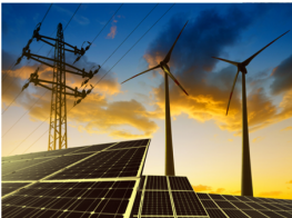
Smart power systems
